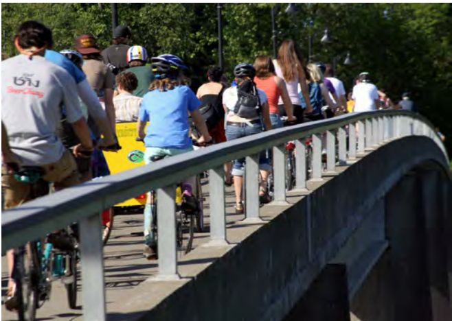
Bridges and other grade-separated crossings provide for critical walking and bicycling connections.
