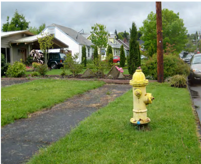
Missing sidewalk segments can make walking much more difficult.
